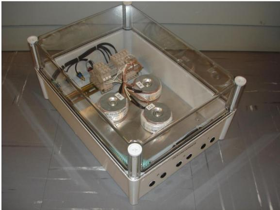
Figure C-2: Voltage instrument transformer
